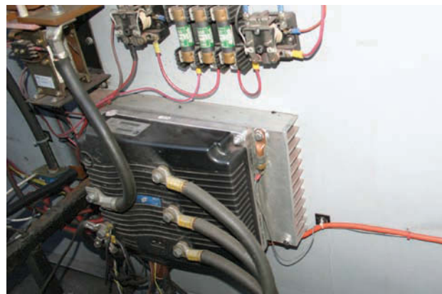
Figure 4 The Curtis ac-motor controller gives 80 hp with the battery/motor combination.
